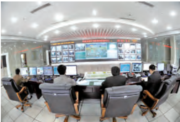
Digital control center
