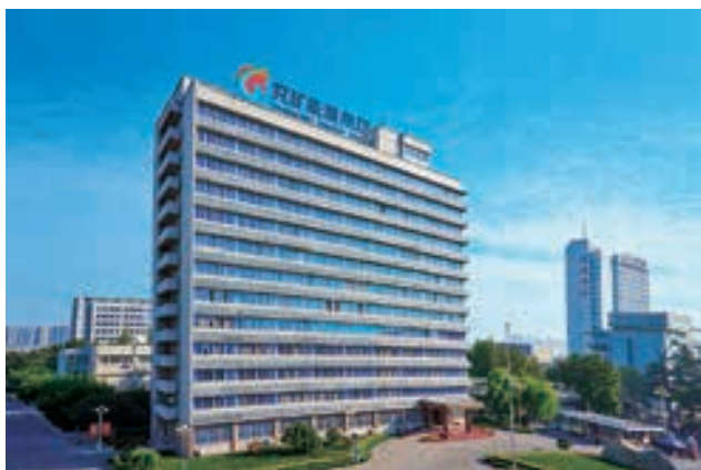
Yankuang Energy Building
