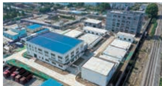
Nantun Coal Mine: High-Salt Wastewater Treatment Project
