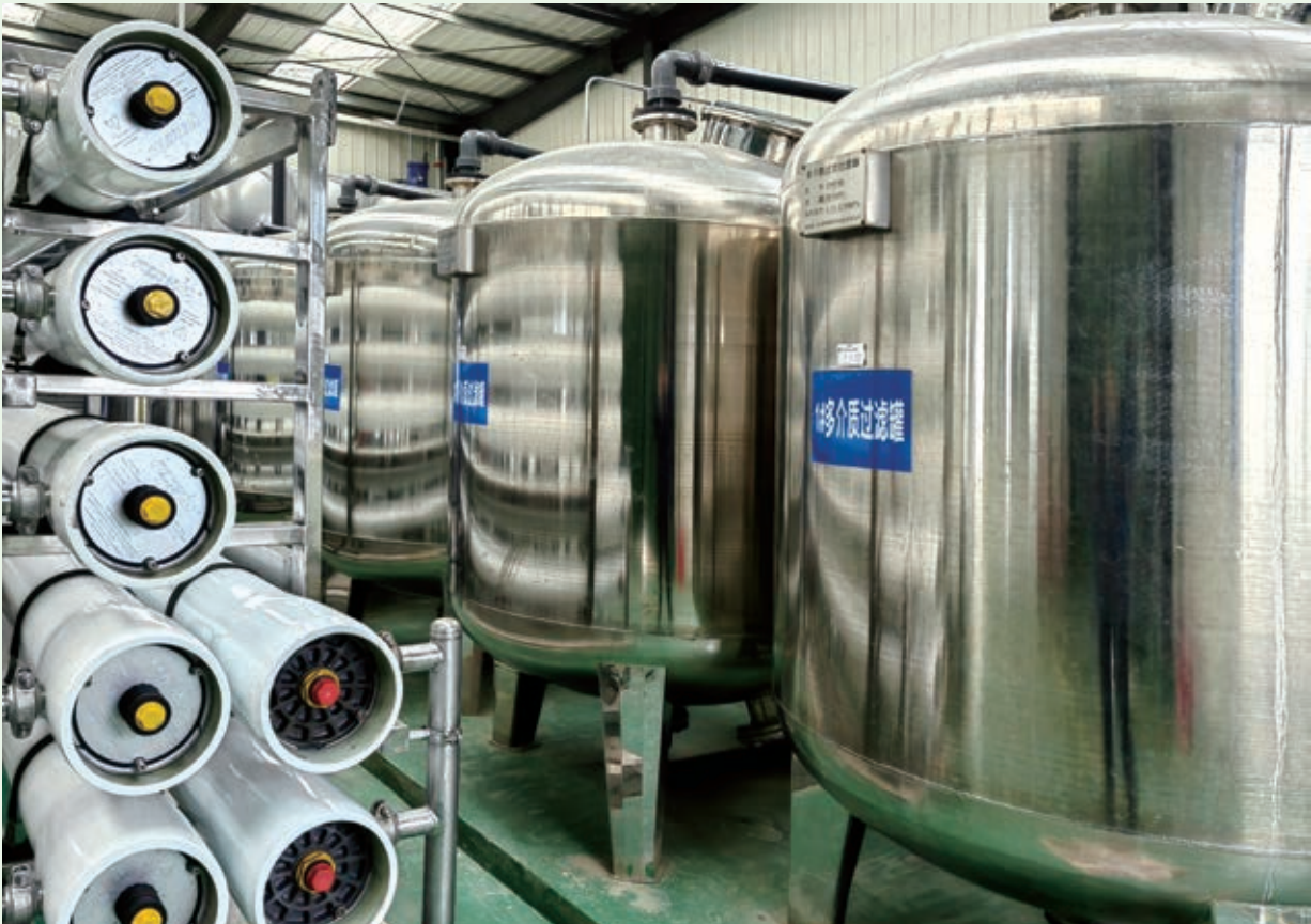
Jinjitan Coal Mine adopts deep treatment system for mine water
